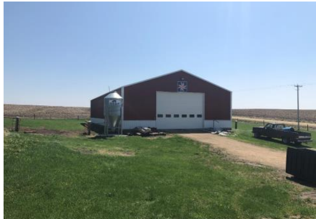
45 x 90 Machine Shed. View from West.
