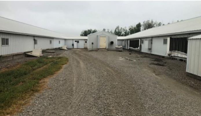
Load-out & Wean-hold Nursery
